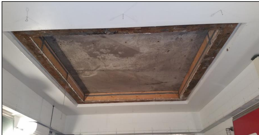
Receive Room View of Test Specimen Installation
